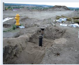
New Water Main Installation
