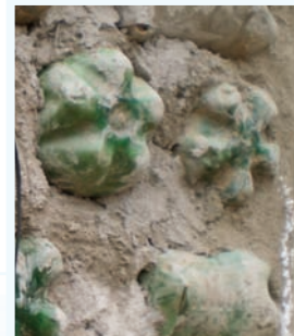
bricks made with mud-filled soda bottles
