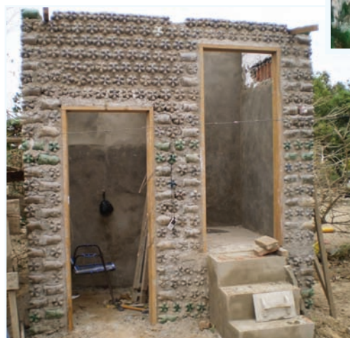
New baños structure
